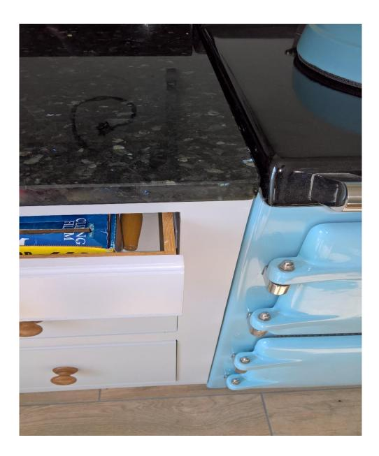
A neat installation, show the front fill piece has been blended in and the work top fitted with about 3mm gap.
