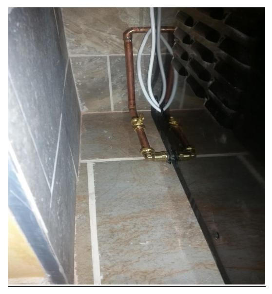
Picture show gas fittings, note the electric flexible cables at the back.
