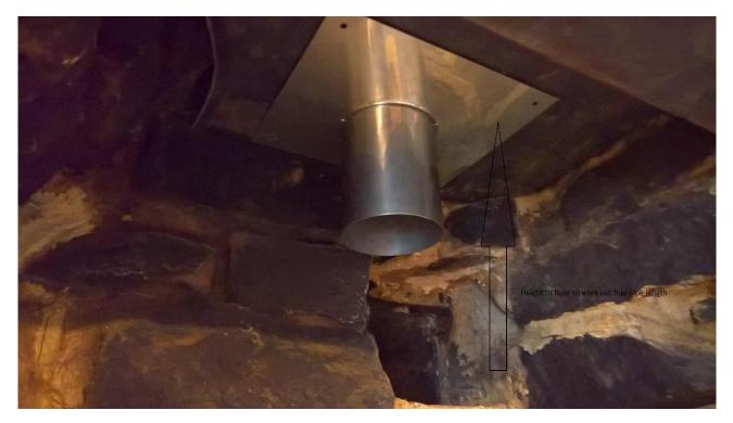
This is a picture of a register plate adaptor, the gloss black vitreous enamel flue pipe slip over it. When installed, please email the distance from the plate to the floor as shown, so we know what flue pipe to bring. The centre of the flue should be 120-125mm from the finished back wall.
