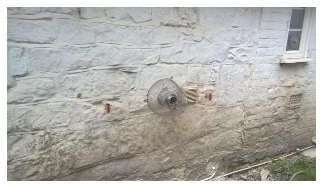
Picture shows oven vents, main exhaust vent, air inlet and second oven vent on balanced flue model.
